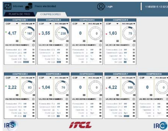
Figure 5.16 - IRS, industrial refrigeration supervision
